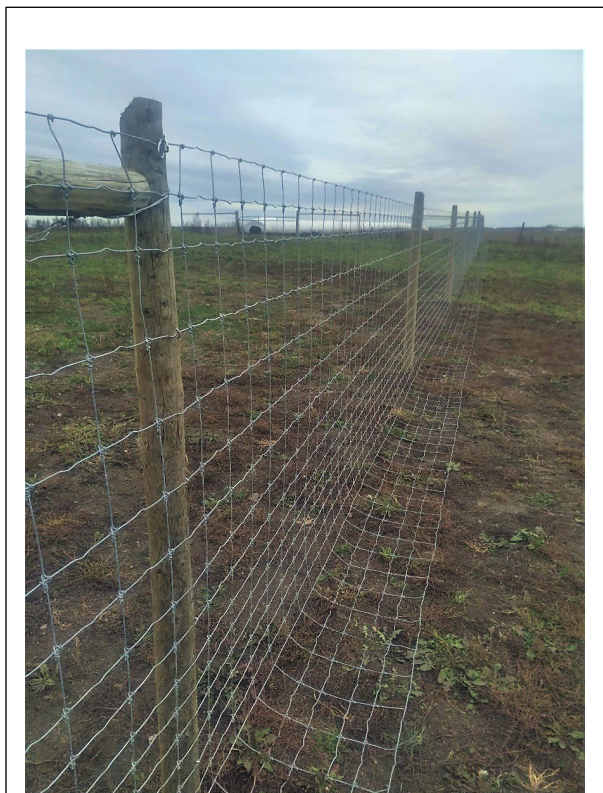
Fixed-knot fence with apron to deter burrowing
