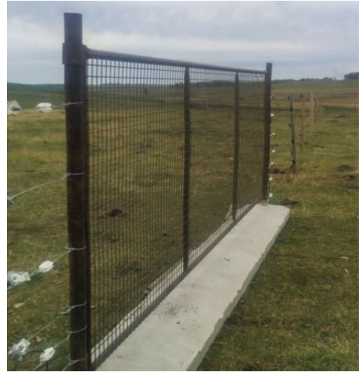
Gate with concrete threshold
